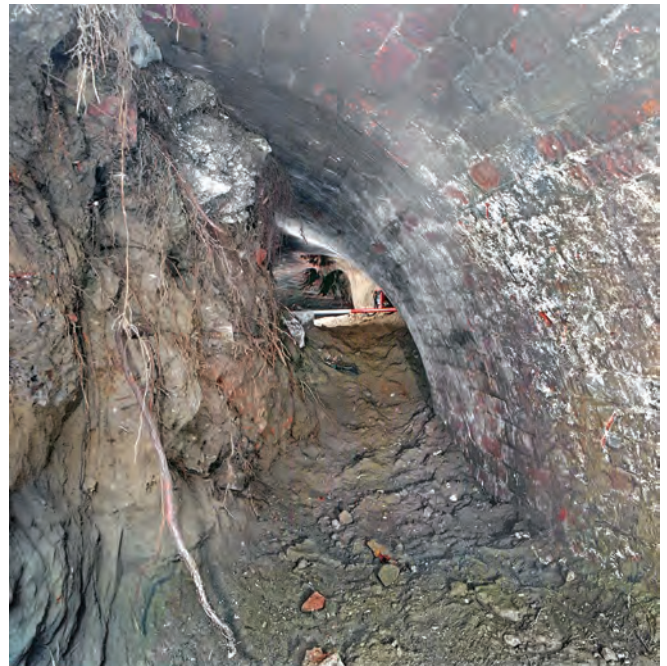
Looking west into the tunnel system from the entrance.
